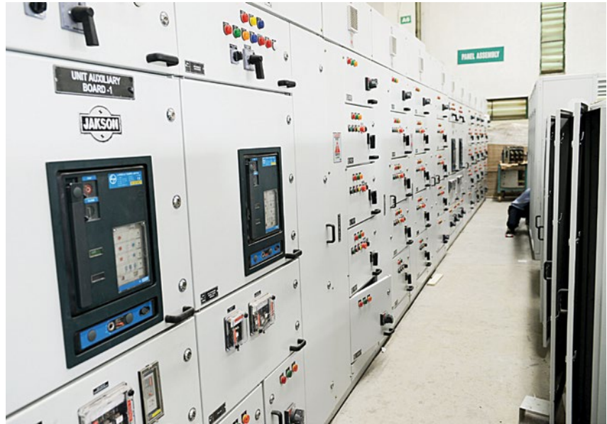
Control panel and switchgear unit at Greater Noida
