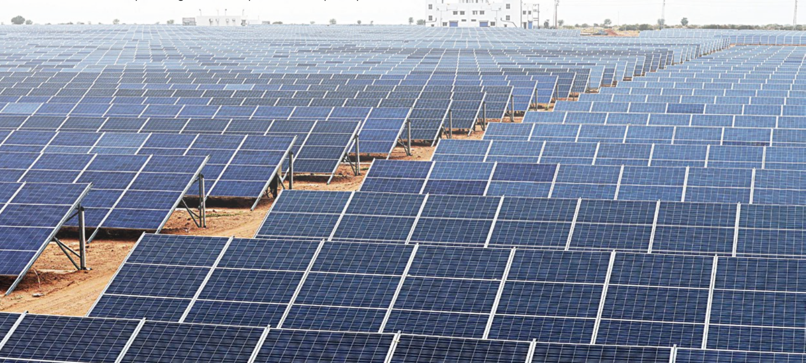
Jakson solar power generation plant at Baap, Rajasthan
